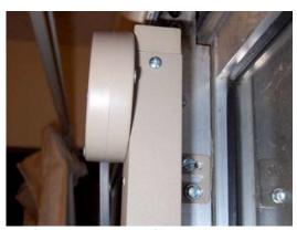
4th hex head screw installed on top mounting bracket
