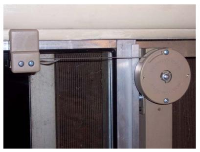
The door closer mounts on the inside of the door (inside the house), on the moving panel on the side opposite of the door handle. The tape anchor is mounted to the door frame, 6" toward the handle side of the door, on the door frame
