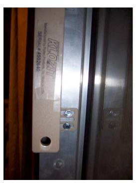
Closer vertical with door and bottom two hex head mounting screws installed on mounting bracket
