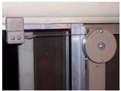
Strap closer correctly installed on left handed door with strap anchor cover installed.
