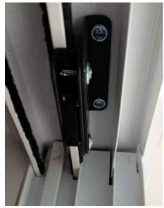
Gravity latch and mounting bracket mounted to under side of top door frame.
