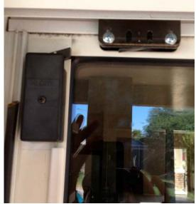
Latch body (left) with cable coming from below, concealed by white plastic cable cover. Latch striker in locked position
