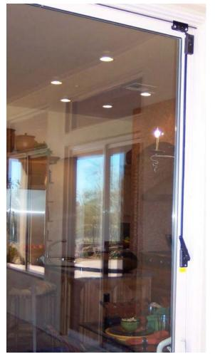
Exterior view of door latch system with Latch handle, plastic cable cover, latch body and gravity latch bracket visible.
